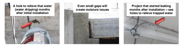
Precast planks are typically made with a denser concrete mix, meaning water that gets into the cavities will eventually come out, but it may take a few weeks or months.
